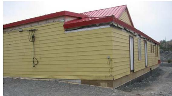
Support posts holding up a portion of the rear roof will be replaced, the perimeter wall on the east side (YK Bay facing) will be replaced where possible with concrete, and a geo-membrane layer placed where needed to prevent water runoff from entering the crawlspace. We thank
