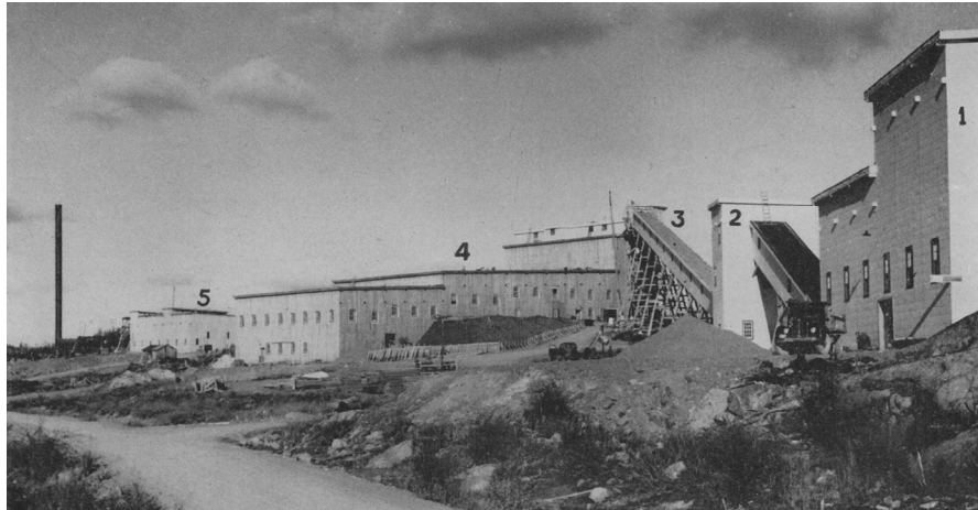
Figure 1: Treatment plant 1948-1949. 1) crusher, 2) screen house, 3) conveyor gallery, 4) grinding and cyanidation plant, 5) original Allis Chalmers roaster and stack.
